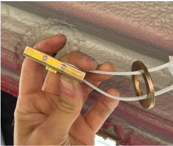
3.1 Insert the anchor head into the hole
