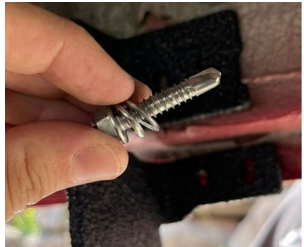
7.2 Insert a 1/4" lock washer and a 1/4" washer onto a #14 x 1.25" self-drilling screw
