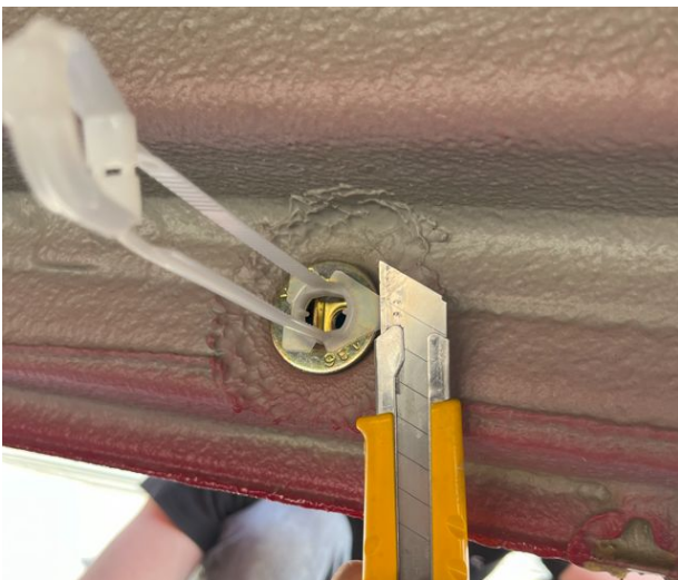
3.3 Cut off the excess strap ends
