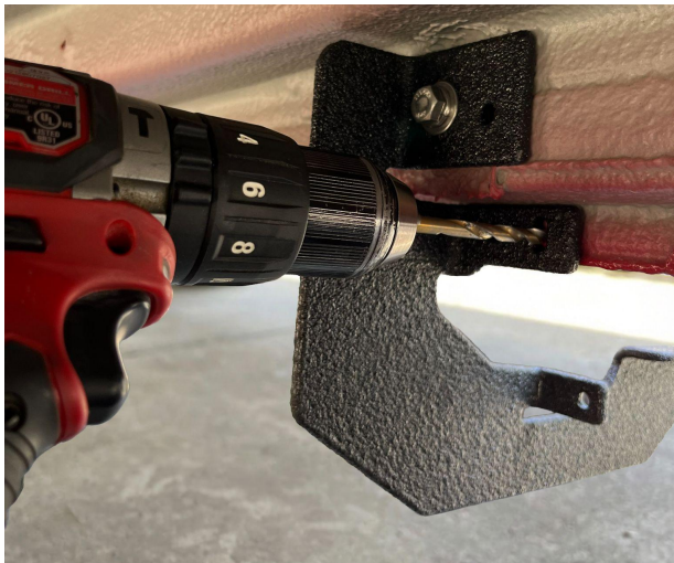
5.1 Drill the vehicle lip using a 1/4" metal drill bit at the center of the lower slotted hole of the brackets
