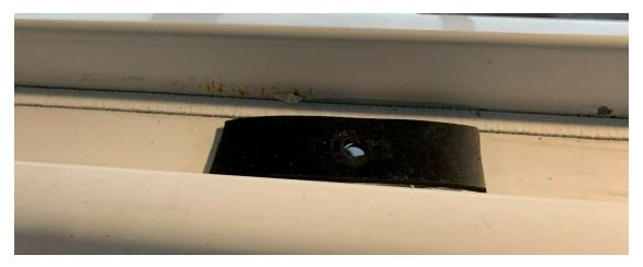
1.7 Apply a 2nd bead of SIKA221 generously (approximately 1/2" bead diameter) around the circumference of the holes in the rubber plates. The joint of Sika221 must be as uniform as possible and seal the circumference of the holes.
