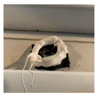
1.6 Place the rubber sheets with their holes aligned as best as possible with the center of the openings on the first bead of SIKA221.
